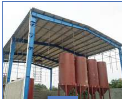
Pre-Engineered Structure of Size 60' X 80' X 35' Height for Chemical manufacturing unit at Hattar
